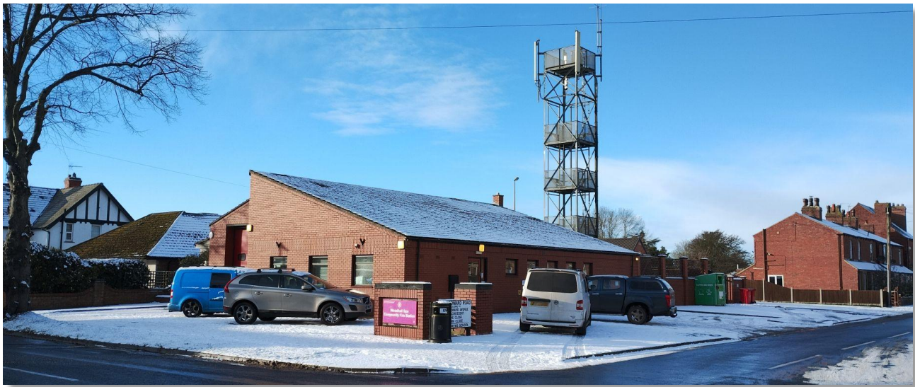
Woodhall Spa Community Fire Station
